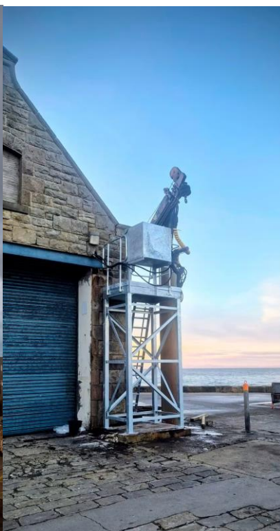
New crane platform
